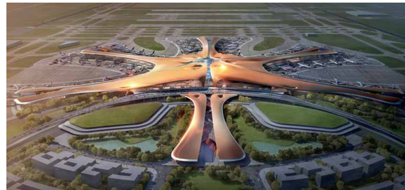
ZAHA HADID ARCHITECTS: Beijing New Airport Terminal Building, Daxing, Beijing, set to become the world's largest airport passenger terminal
